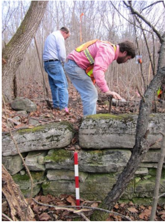
Plate 12: Interior of foundation wall at BbGd-60 (1910085D57)
