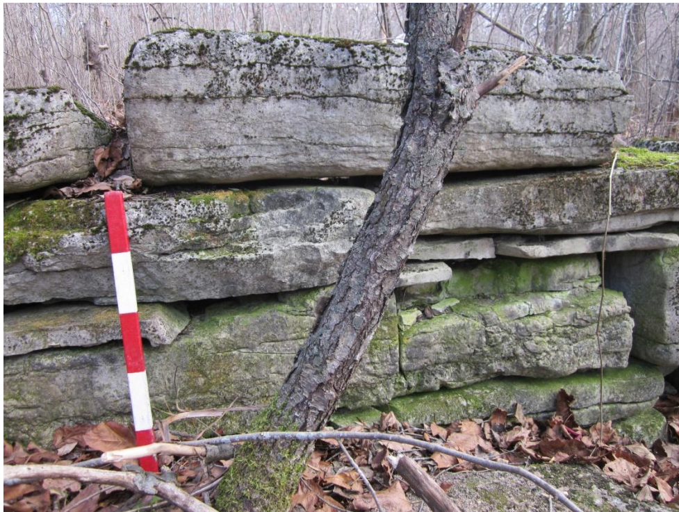
Plate 5: Interior east wall of the foundation (2060101D017)
