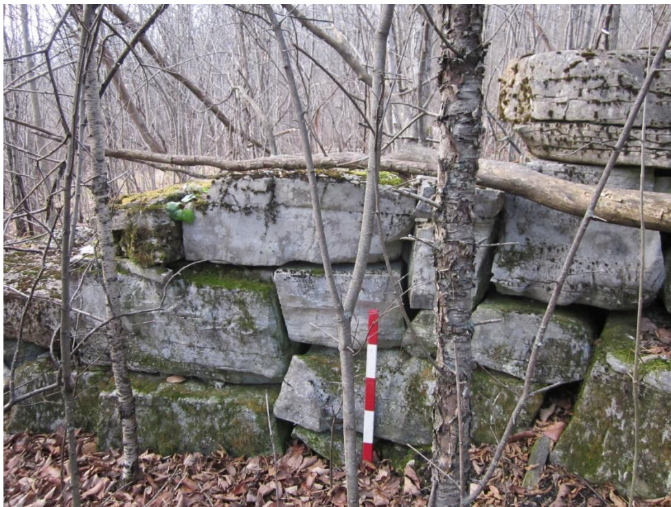
Plate 6: Interior west wall of the foundation (2060101D18)
