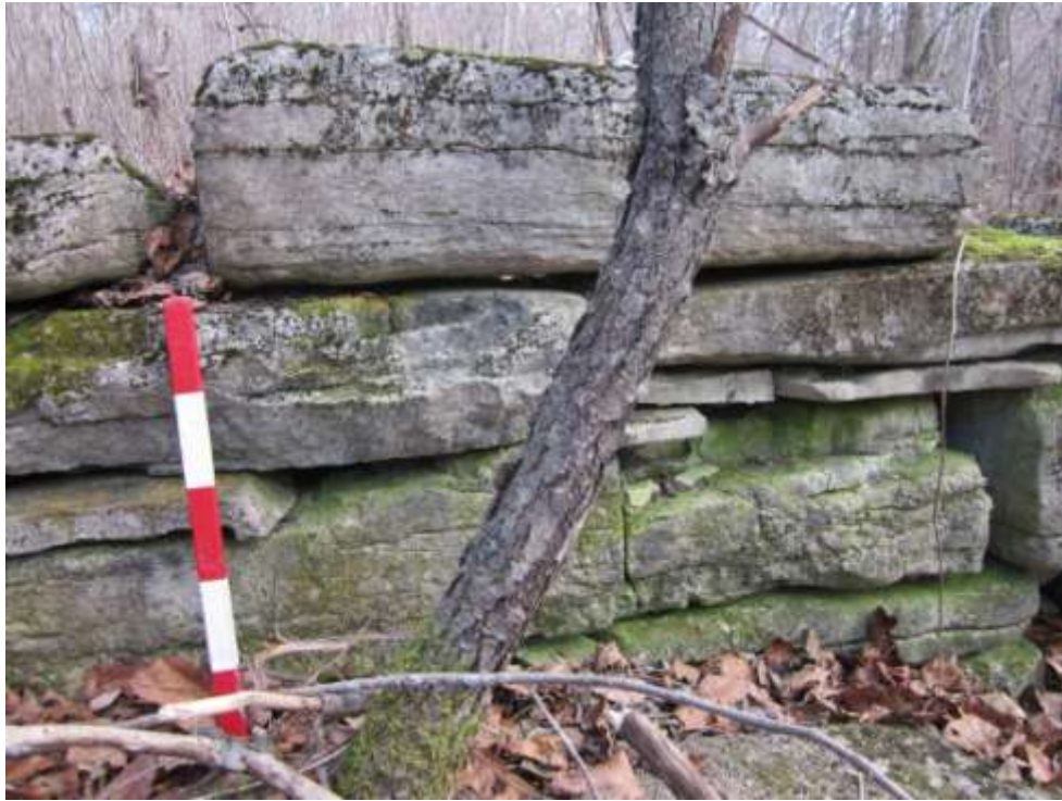
Plate 5: Interior east wall of the foundation (2060101D017)
