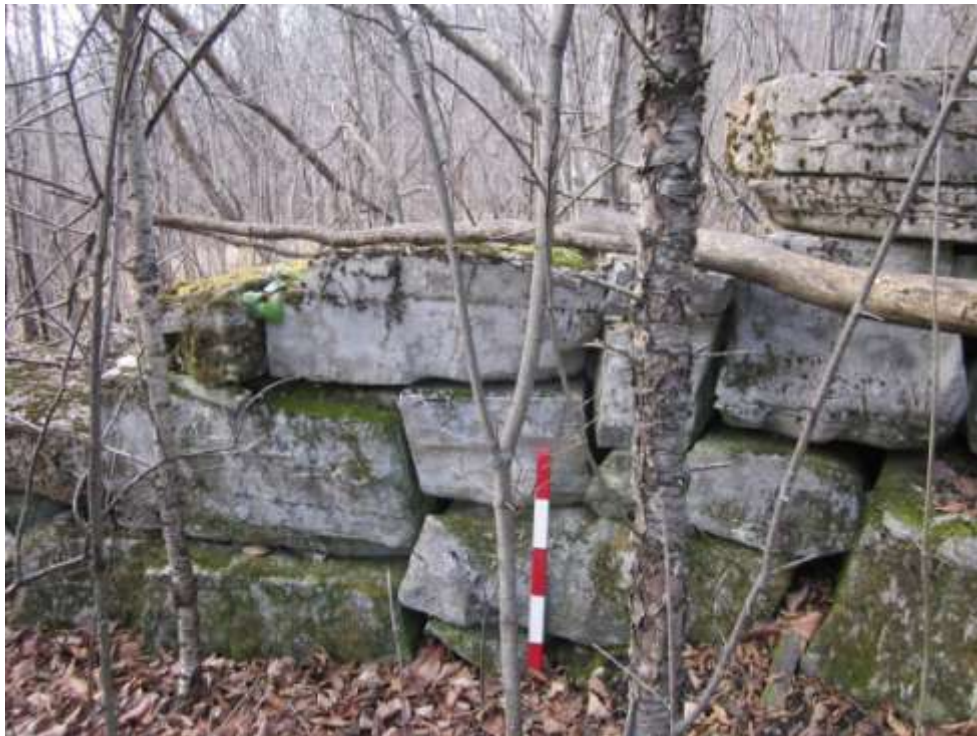
Plate 6: Interior west wall of the foundation (2060101D018)
