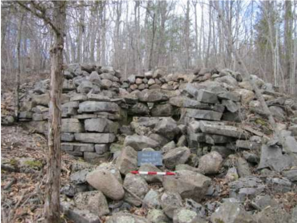
Plate 1: South wall of lime kiln, with draw hole (2060100D01)
