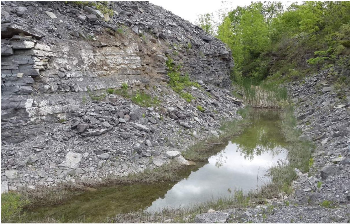
Photo 13: Drainage ditch exiting quarry at the south end (SW3)
