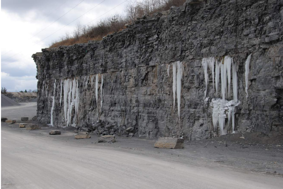
Photo 1: Ice on west wall of south existing quarry, approx. elevation 128 masl, taken Nov. 25, 2013
