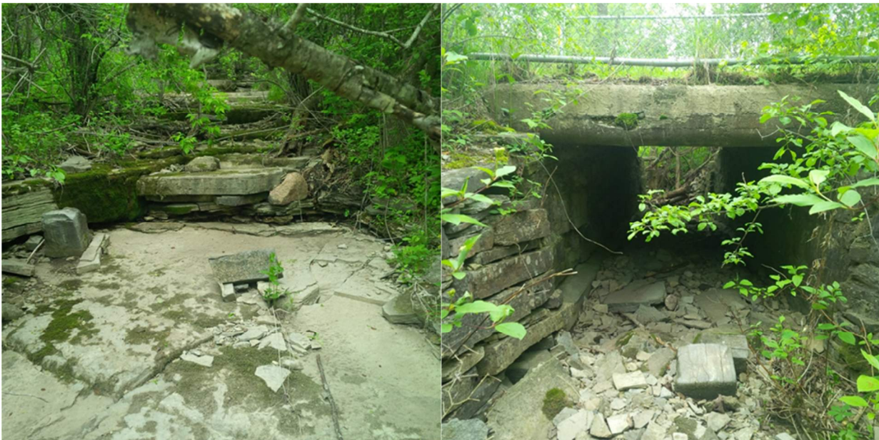
Photo 14: Rectangular culvert under K&P trail (taken from upstream end)
