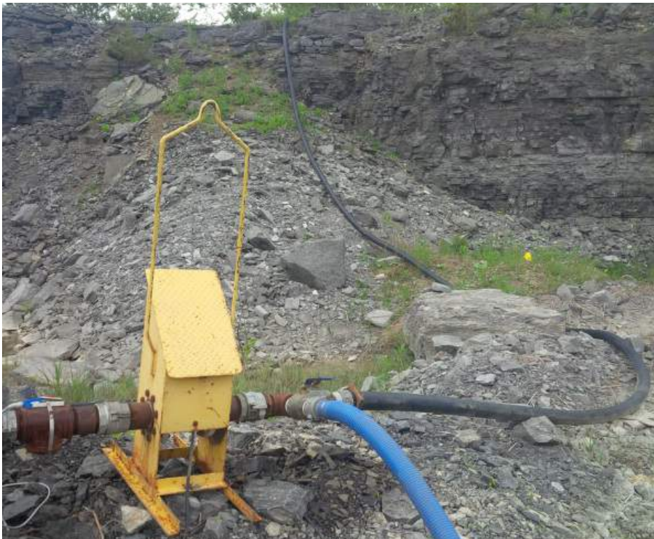
Photo 8: North pump junction. Black pipe goes to culvert and to south quarry (SW1)
