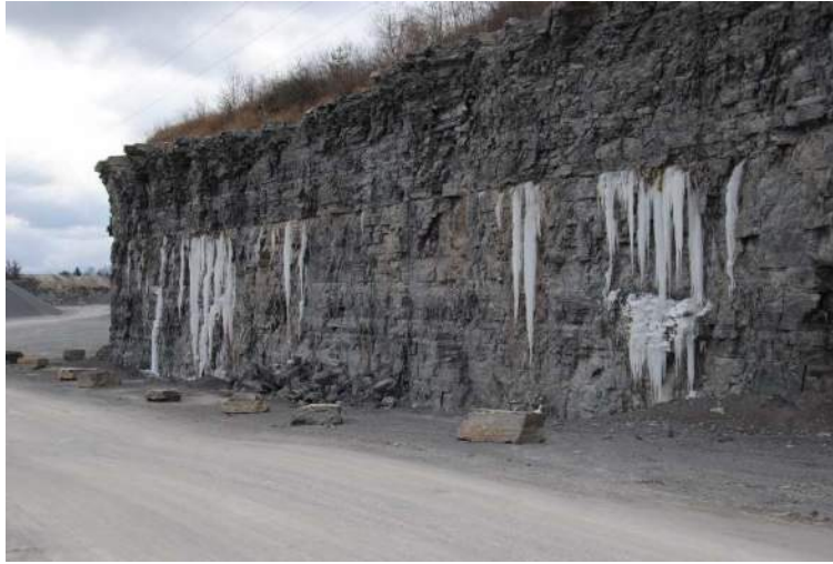
Photo 1: Existing Elginburg South Quarry
