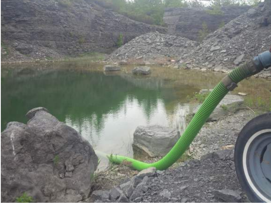
Photo 7: Pumping from the sump of north excavation
