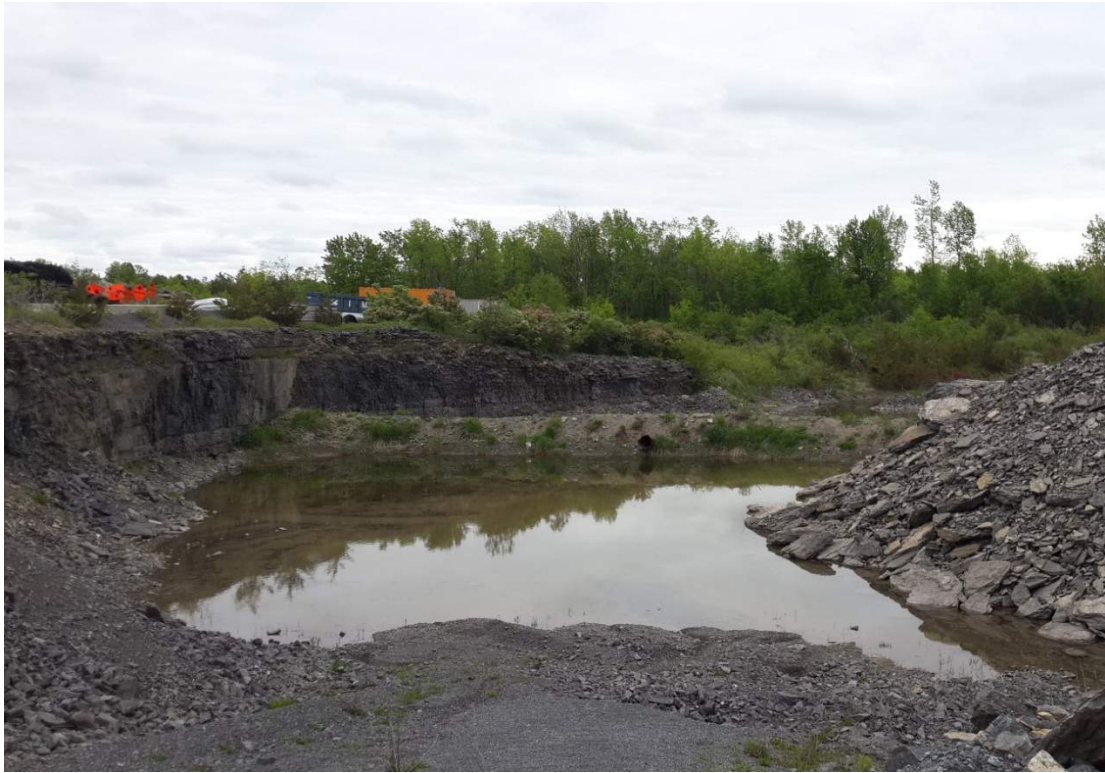
Photo 11: Overflow sediment pond (SW2)
