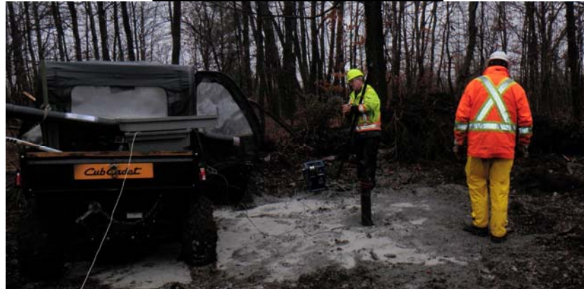
Setting Up System – BH1203
