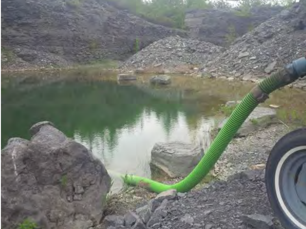
Photo 7: Pumping from the sump of north excavation
